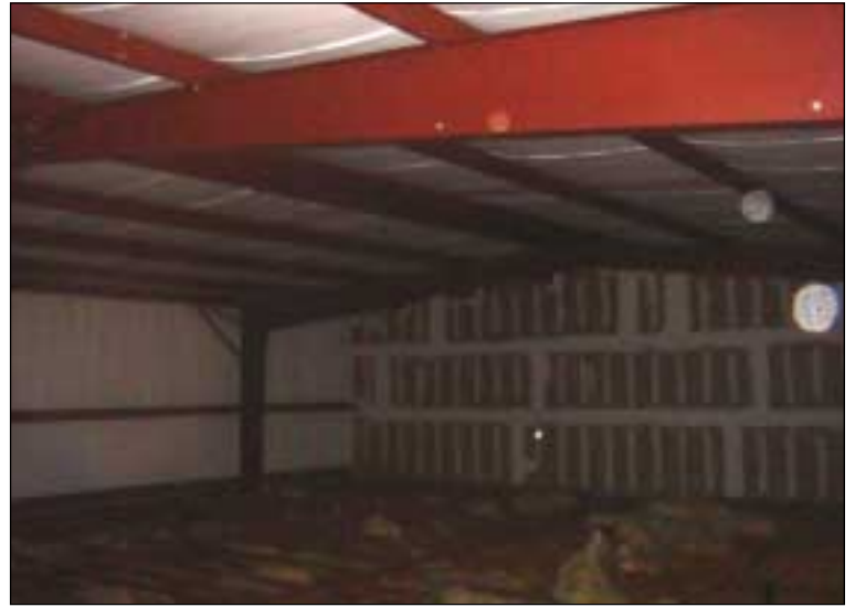
Additional Potential Second Floor Space
